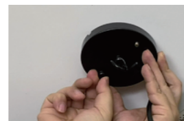
Step 2 Use screws to lock the base to the fixing piece.
